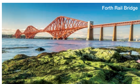
Forth Rail Bridge
